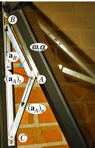
In the mechanism for a window, link AC rotates about a fixed axis through C, and AB undergoes general plane motion. Since point A moves along a curved path, it has two components of acceleration while point B, sliding in a straight track, has only one.
