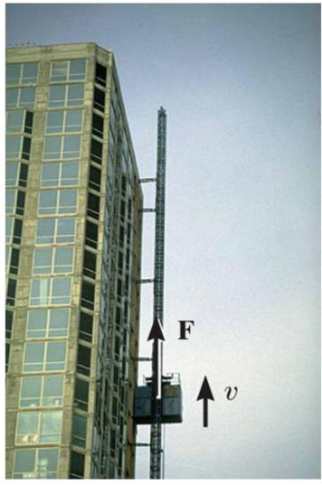
Engines and motors are often rated in terms of their power output. The power output of the motor lifting this elevator is related to the vertical force **F** acting on the elevator, causing it to move upwards.
